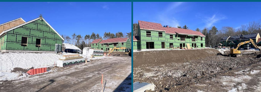
Construction progress at Harriman Hill III, December 2025
